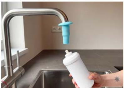
8. Reattach the filter element to the blue primer and turn on the water at a low pressure again.
